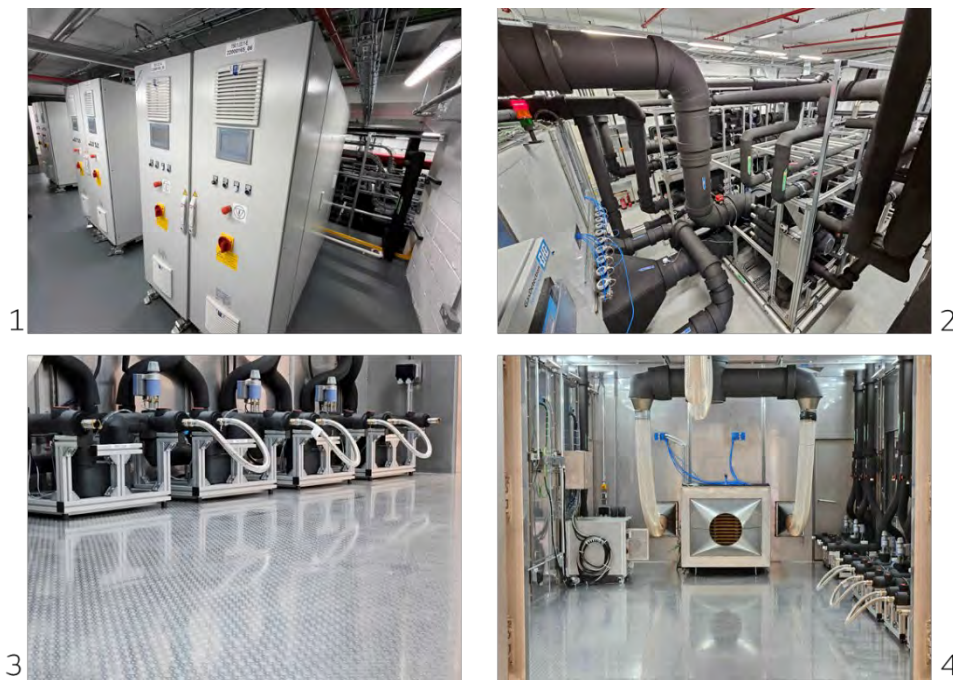
Figure 5: -1: Coolant emulators -2: Plant room -3: Coolant emulators secondary -4: Environmental chamber
